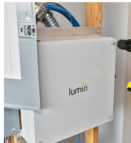
Smart breaker boxes, like the hardware-agnostic Lumin Smart Panel shown here, turn standard panels into smart panels by providing comprehensive energy control and extending whole-home backup.
